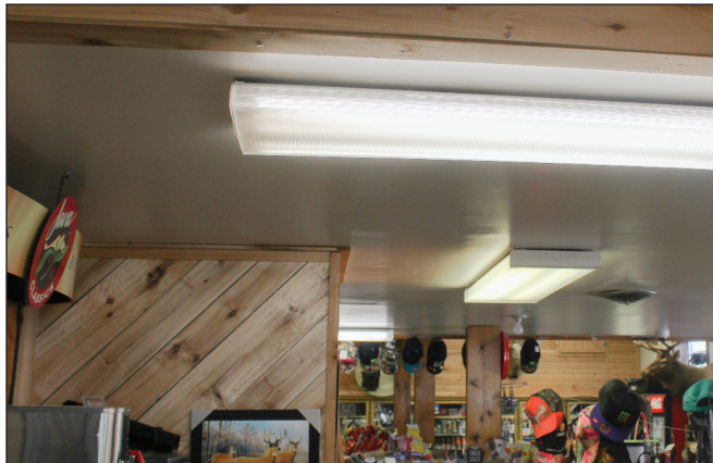
In the foreground is a fixture with new LED lamps, the background has fixture standard T8 fluorescent lamps.
