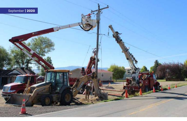
Pictured is Vigilante Electric Cooperative's line crew changing a pole north of Dillon. This pole change was done "hot," so the power was never interrupted to the members off this circuit. | **PHOTO BY ROD SIRING**
